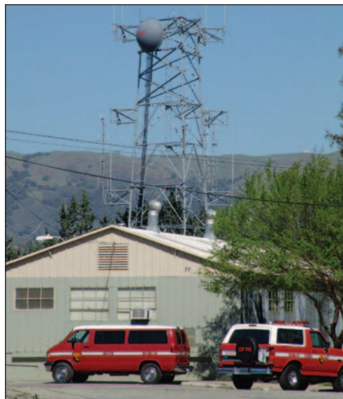
Figure 6. Location that may have serious intermodulation issues
